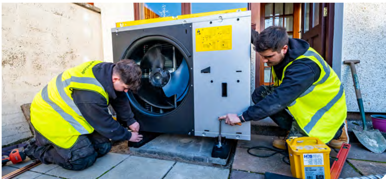
The first Re-Heat heat pump installation underway in Inverness in November 2022
