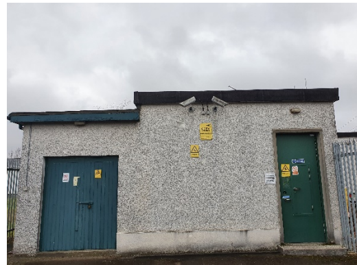
Figure 22 Another example of a typical substation building – Forres.
