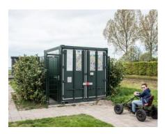
A community battery is large battery, typically 200 to 2000kWh,
