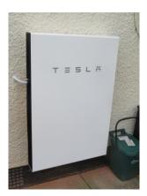
Larger domestic battery systems can typically have a capacity of 5 to 13.5kWh. Some manufacturers have modular systems where the capacity can go up to about 20kWh. The battery can charge from a solar PV system for free, or from
