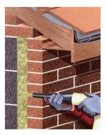
After a tightening of Building Regulations in 1985, it became normal practice to fit insulation in the cavity for new-build homes. Older properties with uninsulated cavities can have insulation retrofitted. This involves drilling regular holes in the external wall and injecting insulating material such as fibre, cellulose, polystyrene beads or polyurethane foam.
